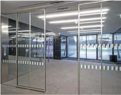
Facade with slim post rail structure seems even lighter and more inviting, and they discreetly and easily blend in with the building architecture. Slimdrive SL NT GEZE particularly hides in glass facades where large door leaves have to be moved and all components have to appear slim and delicate. With its low drive height of only 7 cm, Slimdrive SL NT integrates almost invisibly in the facade and moves door leaf weight up to 125 kg.
